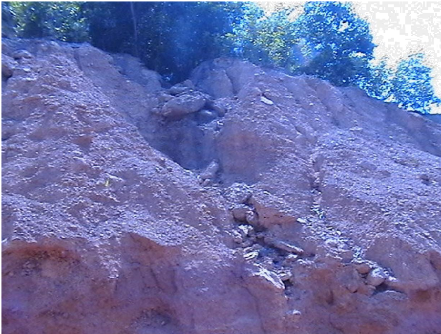
Figure 3.5.5 – Dump Slope Failure and Runoff
